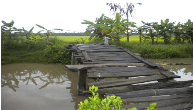
Fig. 2. The wooden bridge built from the 2005's contributions.
